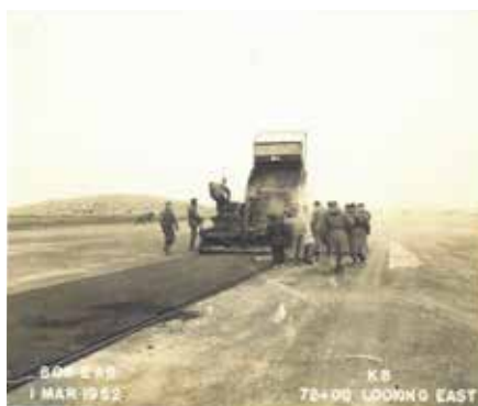
Laying asphalt on a 10,000-foot forward airstrip
