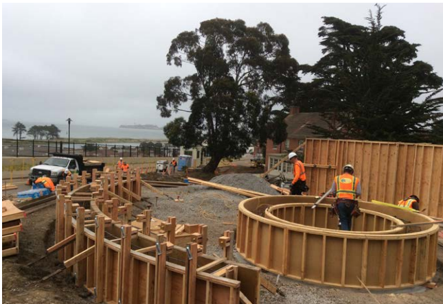
May 6: Building the wooden forms in preparation for pouring the concrete
