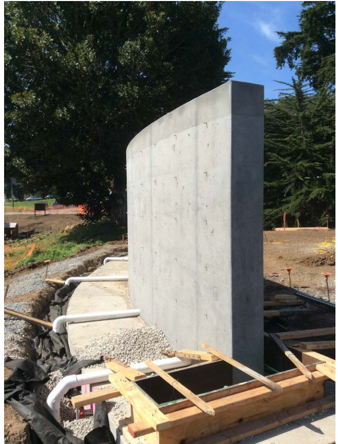
May 19: The wooden forms now removed, the concrete cures and grows stronger in the sun. Once the wall has reached its full strength, the inscribed black granite panels will be secured in place on the concave front surface.
