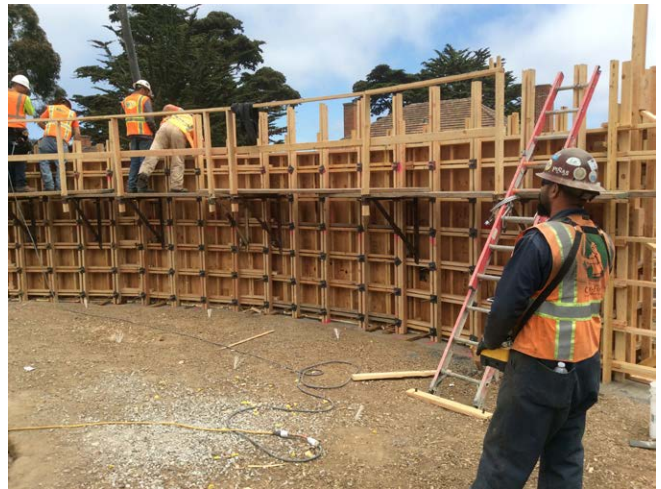
May 11: The crew directs the concrete into the wall form.
