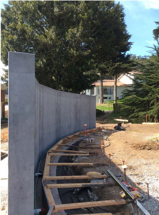
May 19: The wooden forms now removed, the concrete cures and grows stronger in the sun. Once the wall has reached its full strength, the inscribed black granite panels will be secured in place on the concave front surface.
