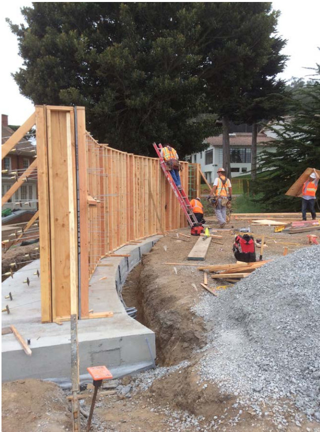
May 6: Putting the last of the wooden form on the main Memorial wall. (In the background is the Monterey cypress tree in memory of Corporal Santiago "Jimmy" Rosas: see story on pages 6 & 7.)
