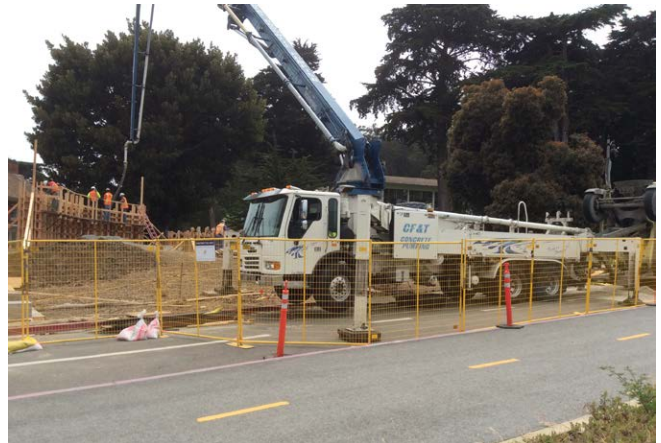
May 11: Concrete is pumped high over the site and down into the main Memorial wall form.
